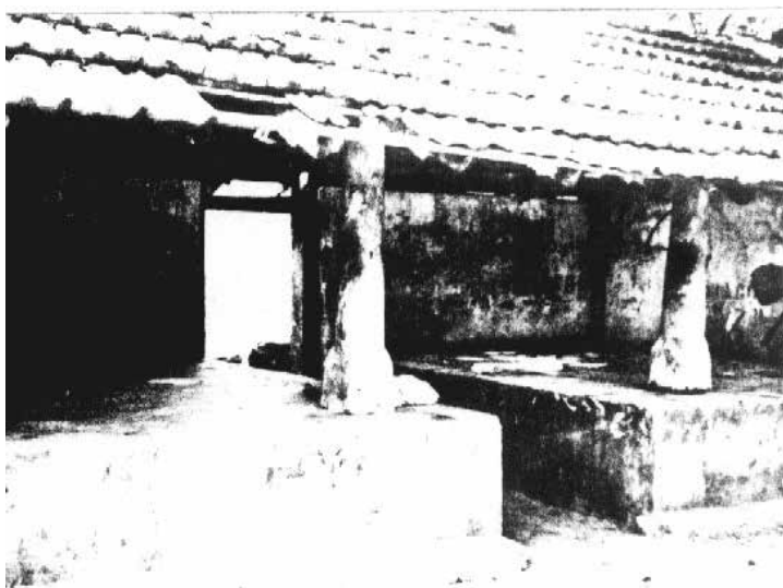
Fig. 11 b - 'Thinnai' at the entrance of the dilapidated 'Poothar Madam' a way side resting place - at Kopay.
