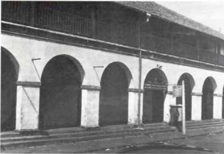
Fig. 5. The Post Office, First Cross Street. This was a draper's, F. X. Pereira's, from 1905 until about ten years ago. The building probably dates from the late nineteenth century.
