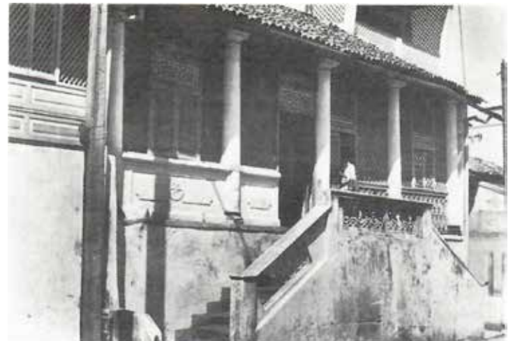
Fig. 14. An early nineteenth-century house in Messenger Street, with coloured lattices incorporating white mal lalis.
