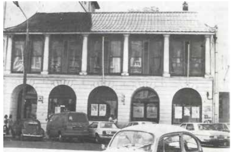
Fig. 4. Air Lanka office, Prince Street. A late eighteenth or early nineteenth-century building in which the arcade and colonnade were probably open originally.
