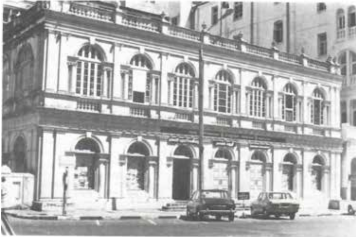
Fig. 2. Ministry of Information, Prince Street.
