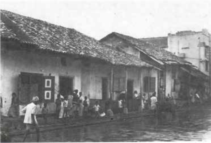
Fig. 9. Houses in Chokku Street, dating probably from the seventeenth and eighteenth centuries.
