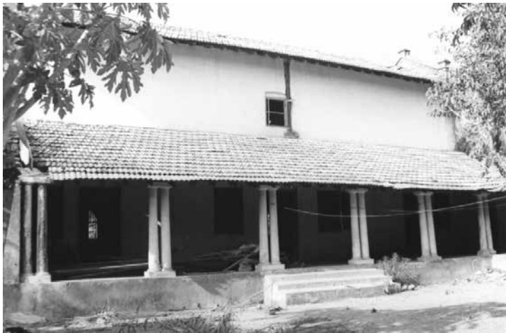
Fig. 7b - A two storied portion of a colonial period courtyard house with gable wall raised above the roof.
