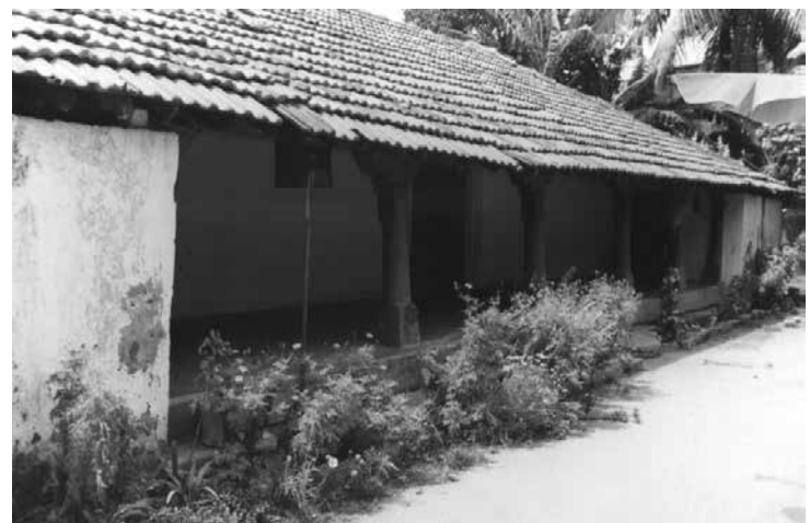
Fig. 12a - Front verandah of a colonial period courtyard house.
